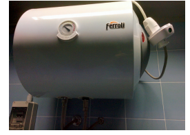
(b) A Water heater equipped with a WeMo Insight Switch.
